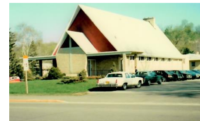
Division Street Church - 1958
